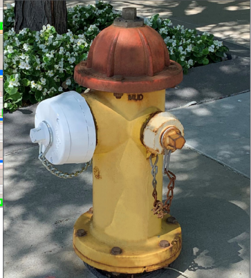
Hydrant with DX node in Downtown Omaha
