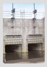
treatment plants, low-head reservoirs and power plants. The side guide seal assembly features an ultra-high molecular weight polymer that positively retains the slide and forms a watertight seal. The frame, slide, stem and fasteners come in stainless steel type 304 and 316, depending on the application. The gate, frame and yoke design conform to AWWA C561 and all seals are factory adjusted and inspected so no adjustment is required in the field.
