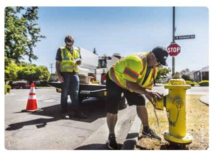
the pilot, and EchoShore-DX sensors were recommended as the technological solution for the project. The acoustic sensors, embedded into hydrant caps, capture acoustic sound waves travelling through the pipe and use the resulting data file to correlate leak locations.
