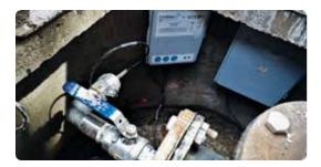
miles of the city's pipe network, with daily leak monitoring scheduled for the next three years. Not only will this non-intrusive leak detection platform notify PUB of a leak or anomaly, it will also monitor advancement of those leaks. This will result in significant savings of valuable resources such as manpower and time, by reducing need for routine site inspections.
